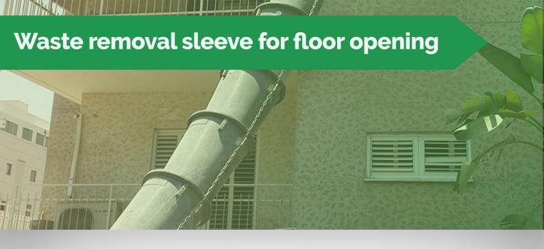
This type of sleeves has to be installed in the beginning of every floor, allowing easy evacuation of the waste during the renovations or construction works.
